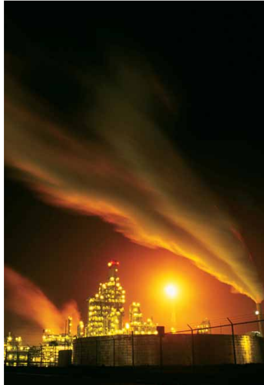
Pictured above: Oil refinery in New Sarpy, Louisiana © Les Stone/Greenpeace
