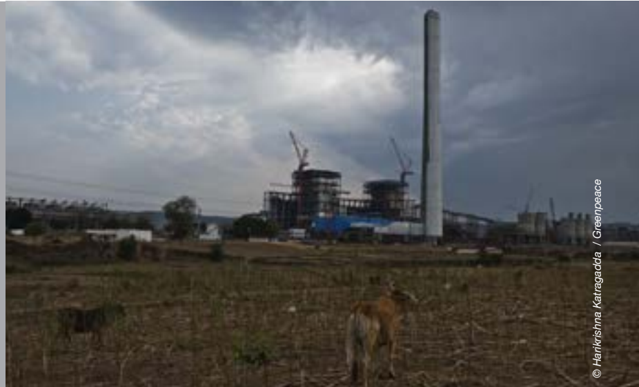
Essar power plant, Singrauli, Madhya Pradesh.
