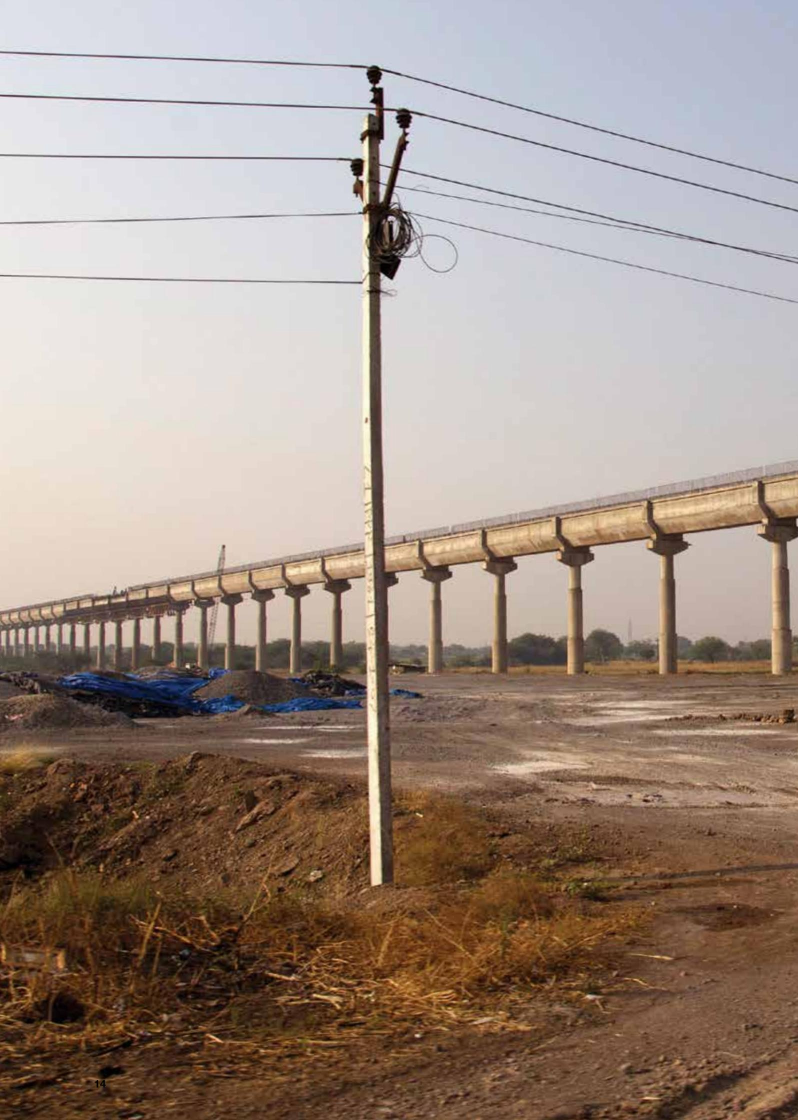
**image** Water Pipeline for a Power Plant Being Built in Solapur An over-bridge for pumped water supply being built in Solapur town, which will carry water to the NTPC power plant from the Ujjani dam in Maharashtra.
